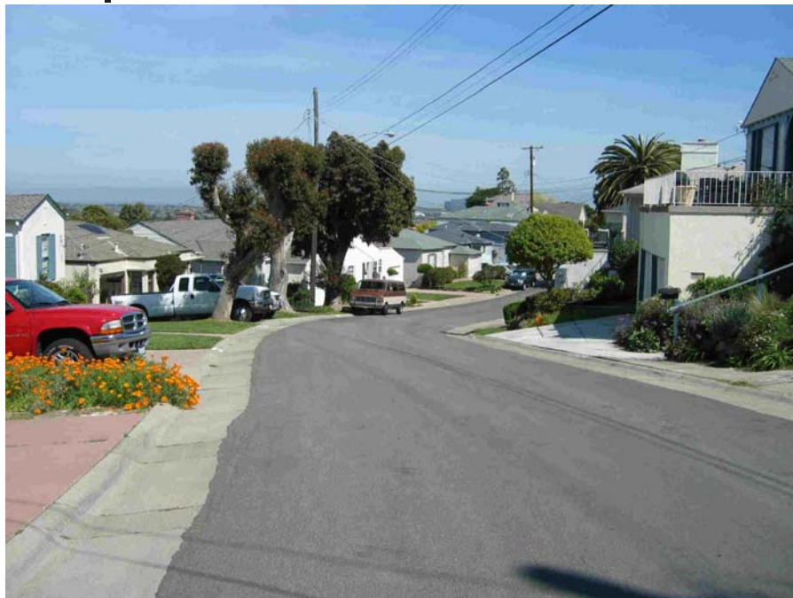
Typical California urban stormwater conveyance system – Street gutter Water & pollutants efficiently moved to creeks
