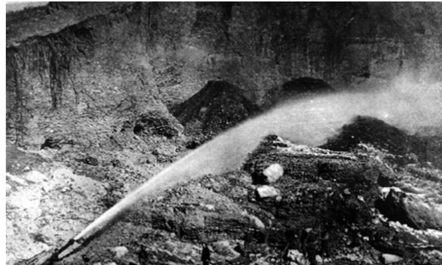
Hydraulic mining, Placer County, CA
