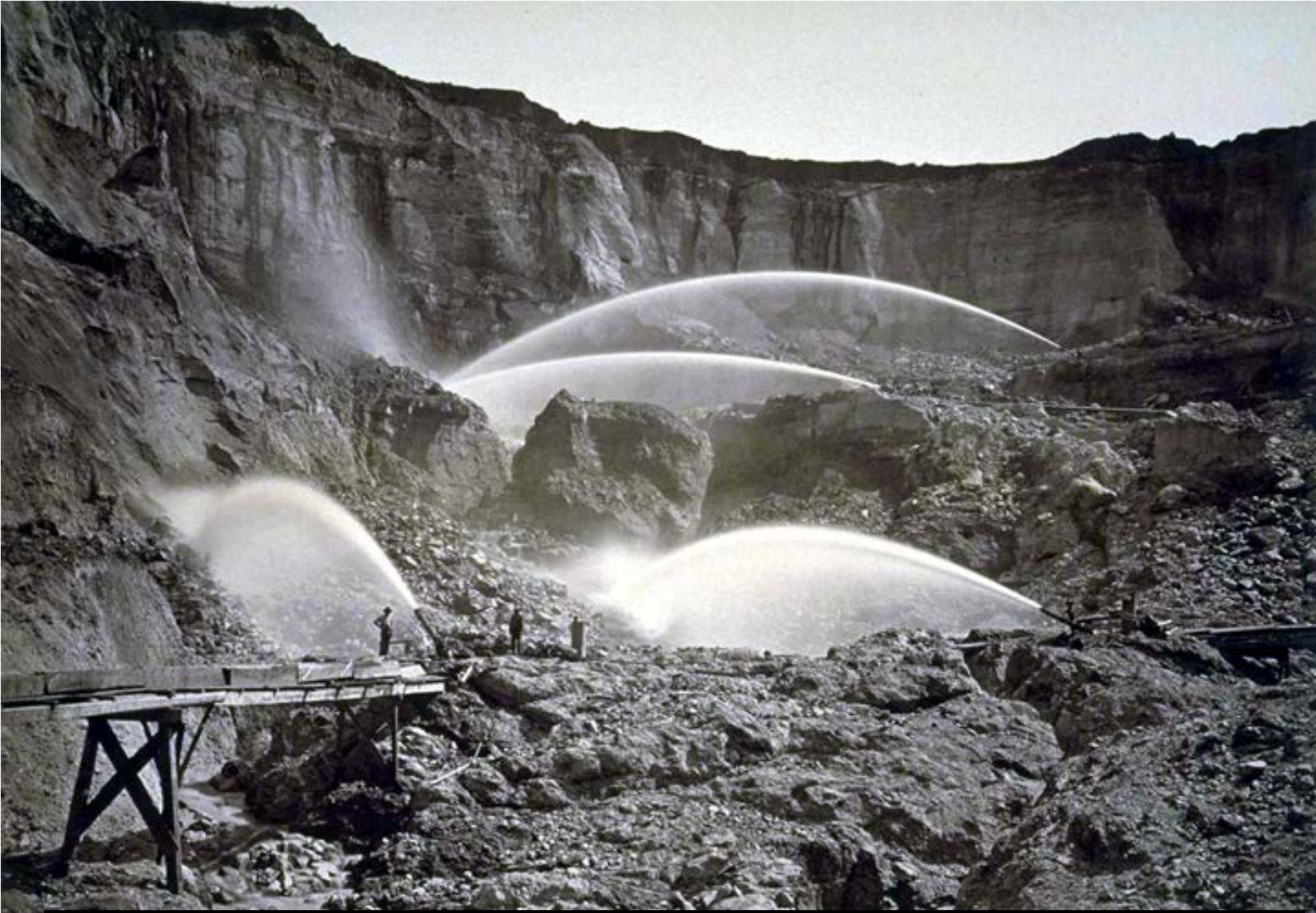
Hydraulic mining, Malakoff Diggins, Nevada County, CA, circa 1880
