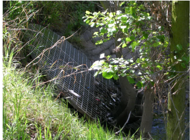
Figure 2. Storm drain at Guadalupe River
