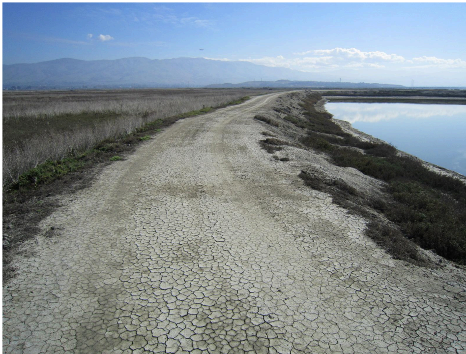
Figure 27: Levee, Santa Clara County. Sarah Pearce, SFEI.
