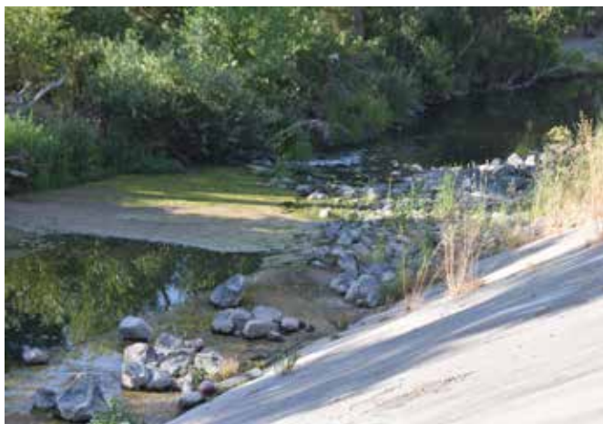
Figure 49. Riprap forming riffle at top of reach; riffle at bottom of reach under Bernal Avenue bridge.
