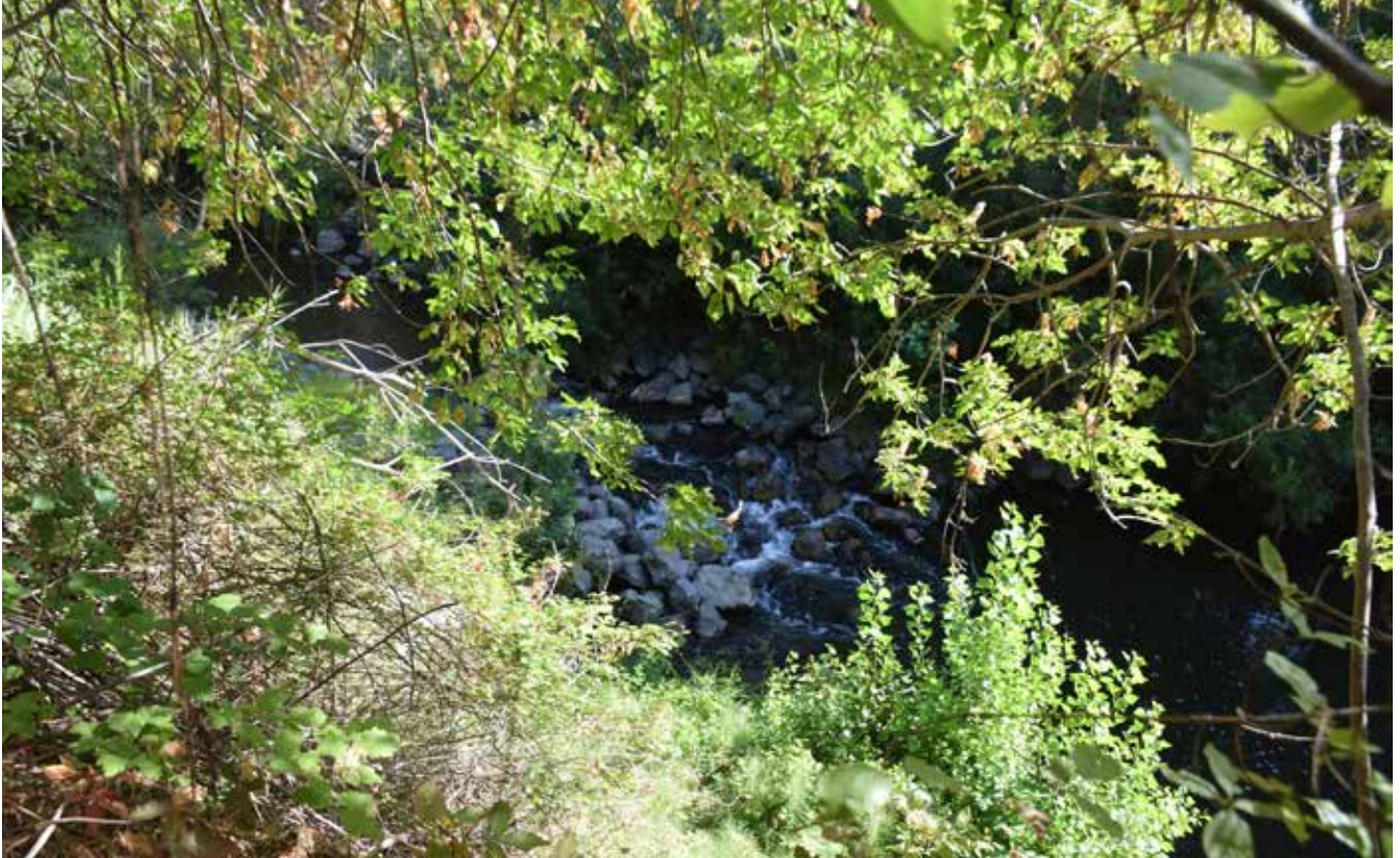
Figure 43. Riprap placed on bed at pump station.
