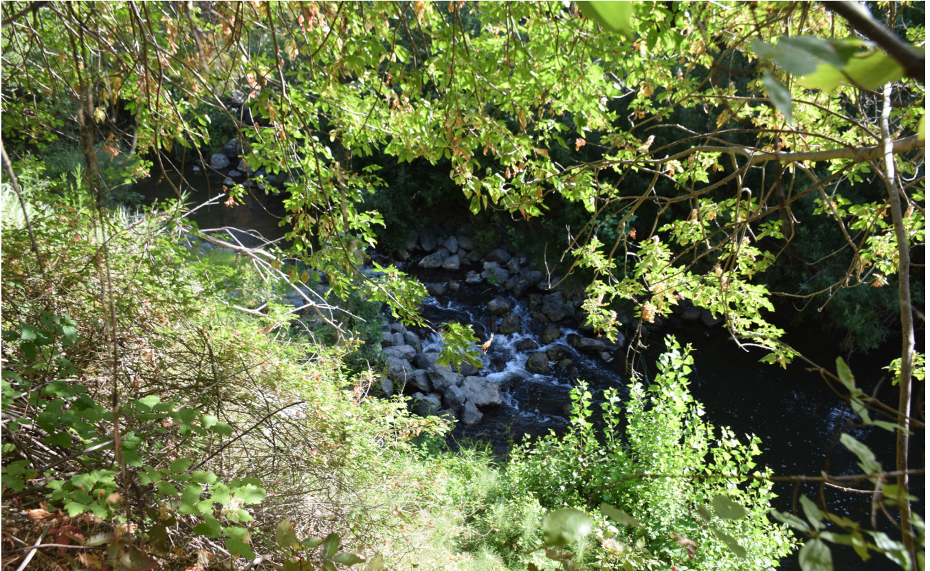
Figure 43. Riprap placed on bed at pump station.
