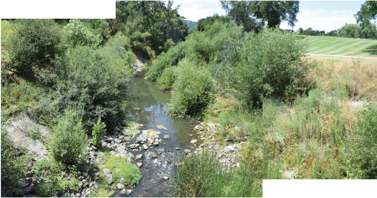
Figure 33. Current view of weir location, looking upstream from the pedestrian bridge.
