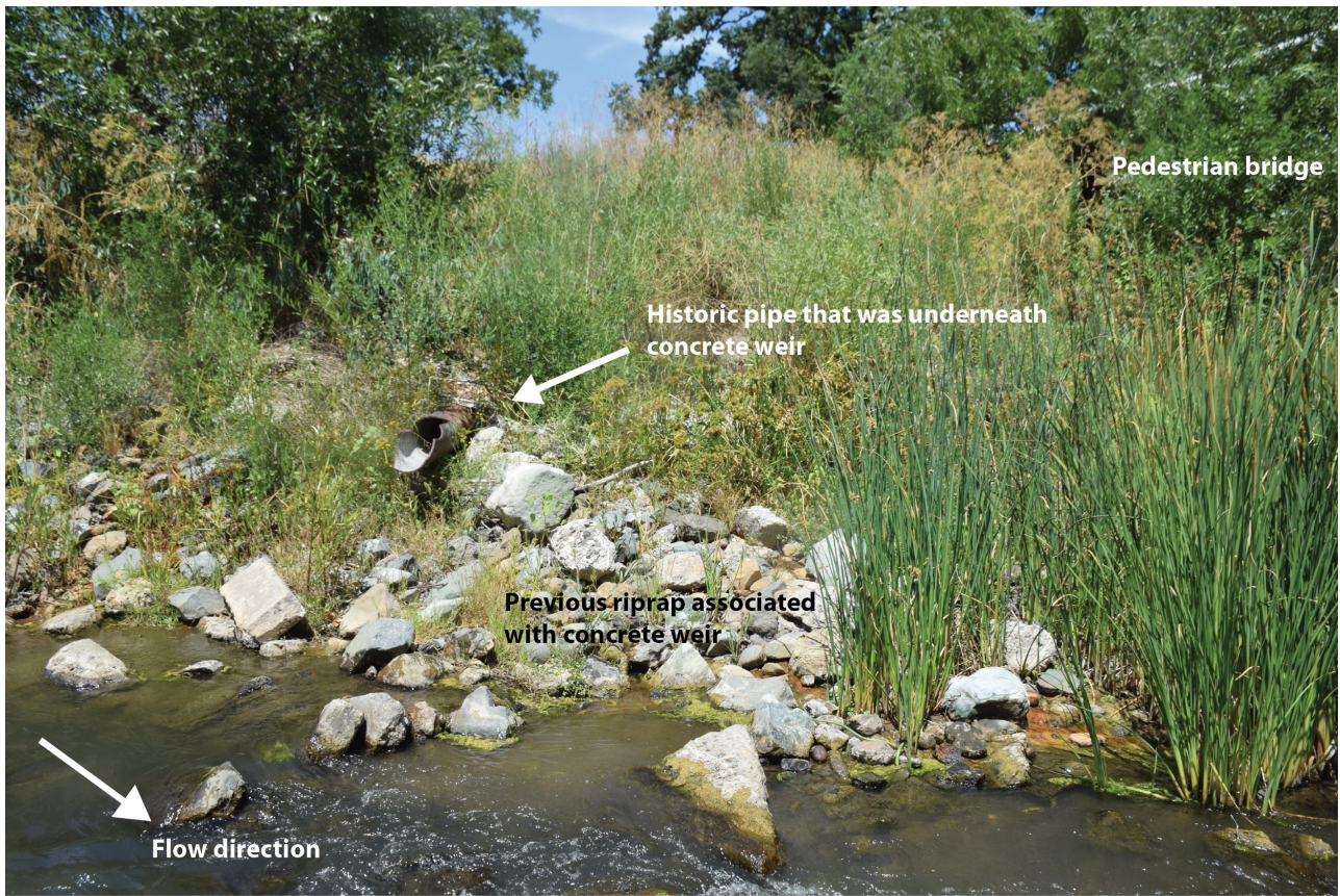
Figure 32. Field photograph of the left bank and an historical pipe that was underneath the concrete weir before it failed and was removed. Pipe is now approximately 1 m above the current bed elevation.
